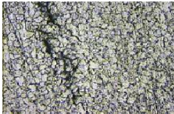
Fig. 7 Microstructure shows cracking (X200)
